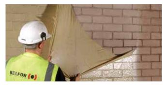
Dry film is removed – along with the soot, dust or other source of contamination – by pulling it off the affected surface.
